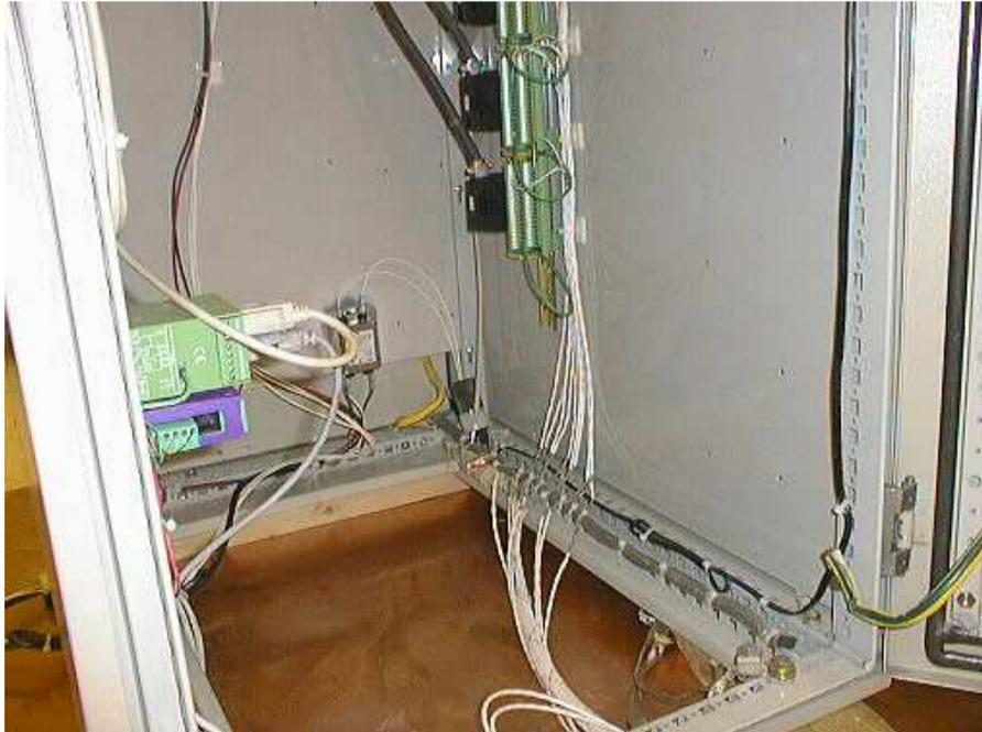
Figure 14-9. Bottom Cable Entry Area
